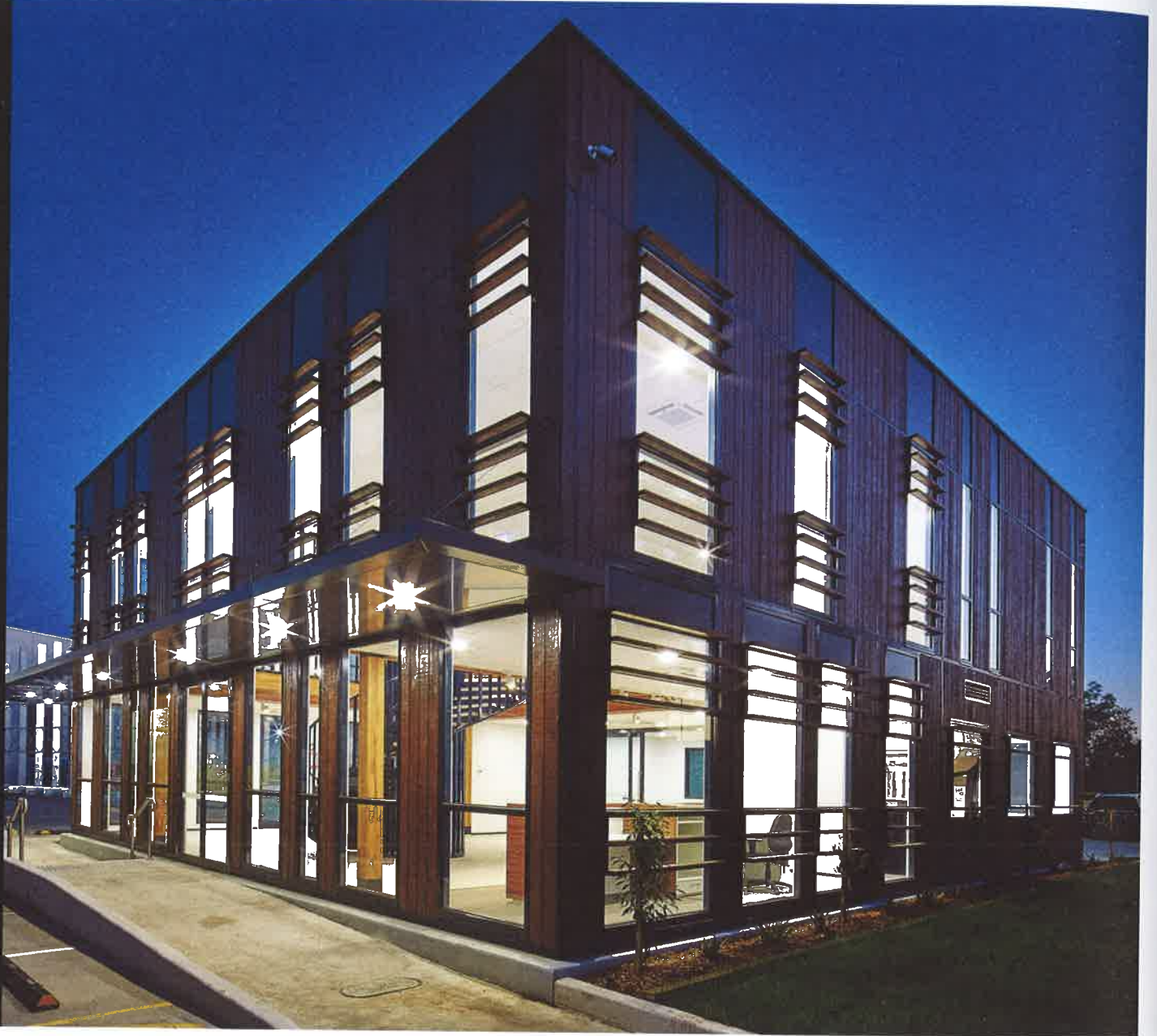
Two storey office assembled on-site in 2.5 days' time (image supplied by Timber Building Systems).
