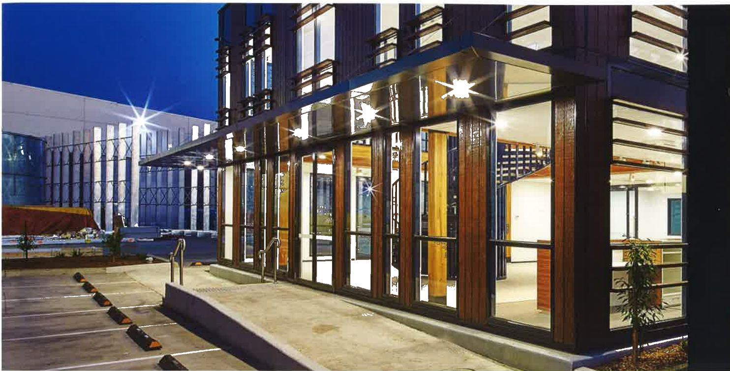
Two storey office assembled on-site in 2.5 days' time (image supplied by Timber Building Systems).
